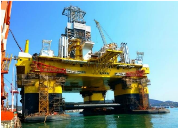
Bluewhale 1 - Year 2016 Oil drilling rig at Quayside in China
