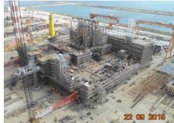
Bluewhale 2 - Year 2015 Construction of Upper Deck Box in China
