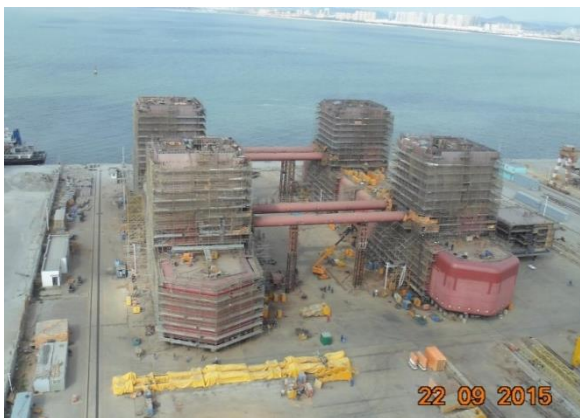
Bluewhale 2 - Year 2015 Lower Hull Construction in China
